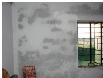
Leaks, damp patches and potholes – sub-standard construction
